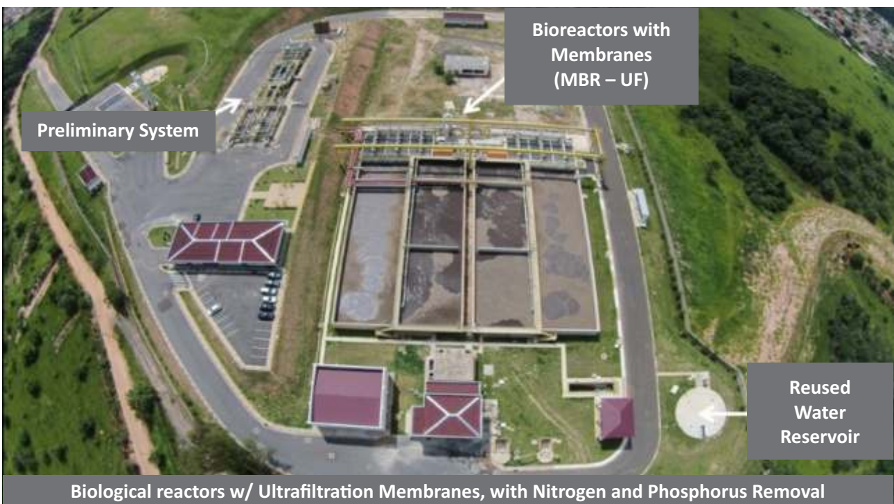
Figure 1. Aerial image of the Water Reuse Production Plant – Capivari II EPAR.
